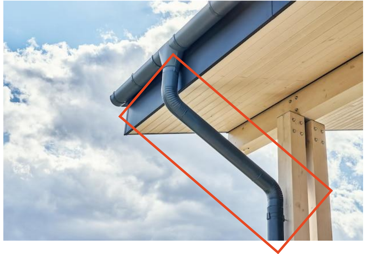
Rainwater Down Pipe
